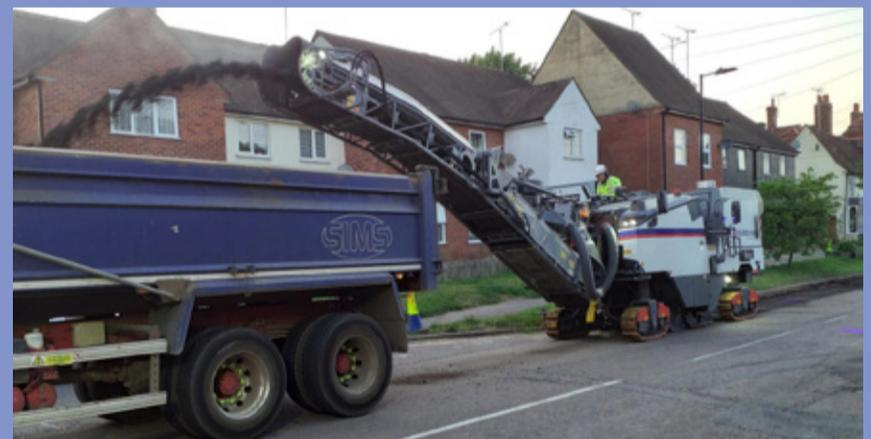
**Insitu-recycling** is only used in limited areas where the road is very badly out of shape. A very durable new surface can be laid, and logistics make it easier to re-use existing materials rather than bring in new stone. It is marginally more expensive treatment per area covered than resurfacing or other treatments."
