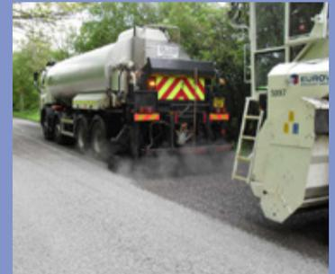
**Micro surfacing** is a slightly more durable and more expensive process which places a thin layer of a completely new surface on the road.
