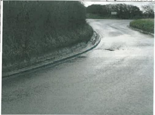
The picture above shows the bend as you approach the turning for Widdington on the road to Newport. The tyre tracks over the kerbed area indicate where vehicles are unintentionally cutting the corner.
