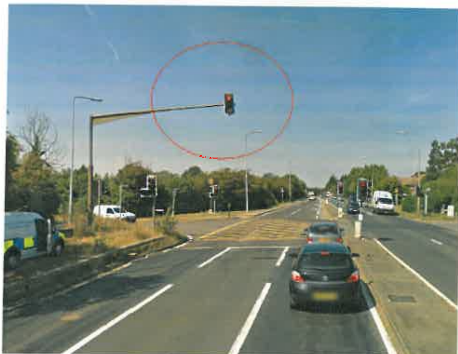
Photo 1 – Example of high level primary traffic signal head used elsewhere within Essex.
