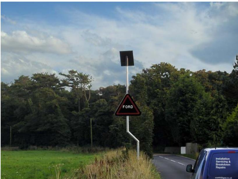
reliable and rugged. It has been in place at Chiswell for four years and there has been a zero failure rate for any of the three signs located there. The company manufacture interactive signs for Caledonian McBain who operate the ferry service to the Hebrides. The signs are manufactured to Highways standards and are certificated to TR2157A and TR2505A.
