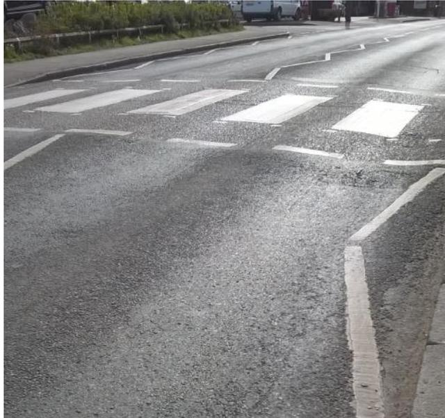
Image 6: View of rutting of existing carriageway.
