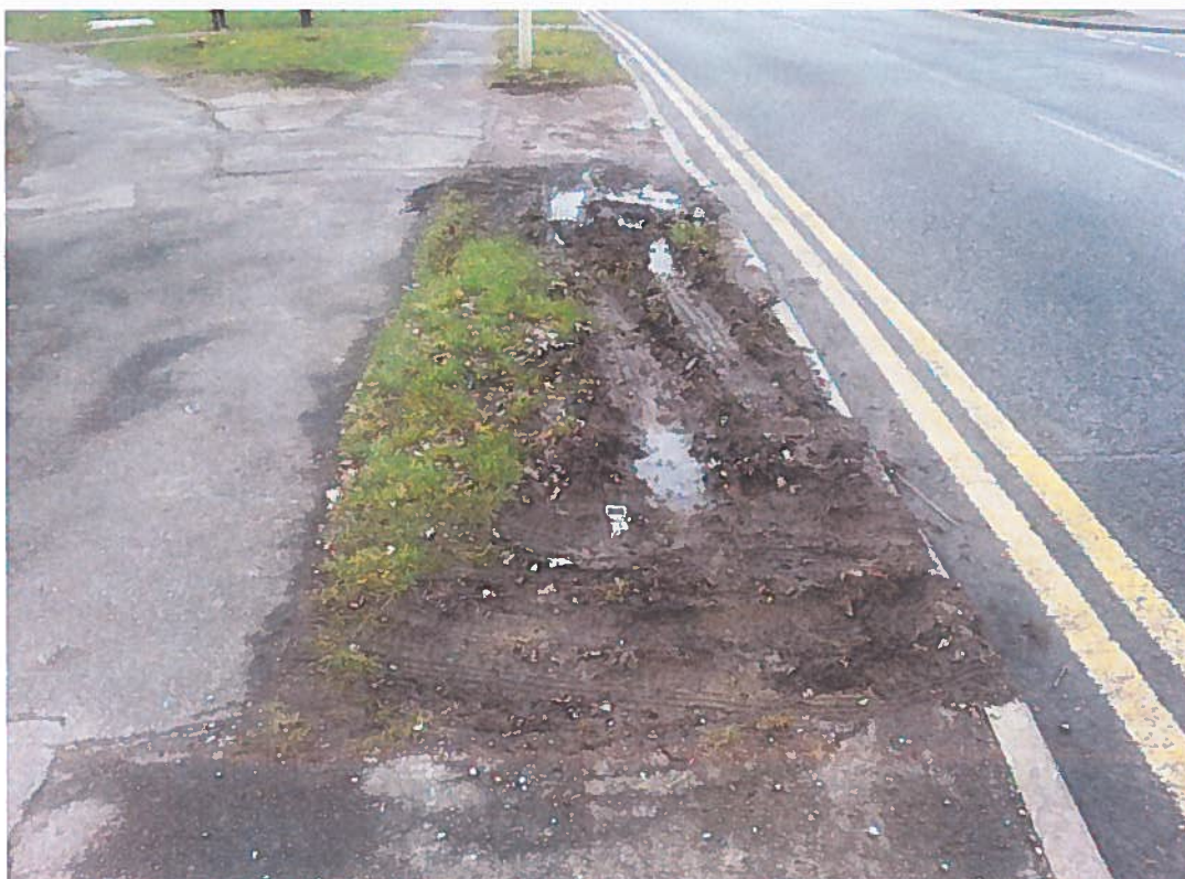
Photo 2 - Rutting in Grass Verge Opposite Woodway
