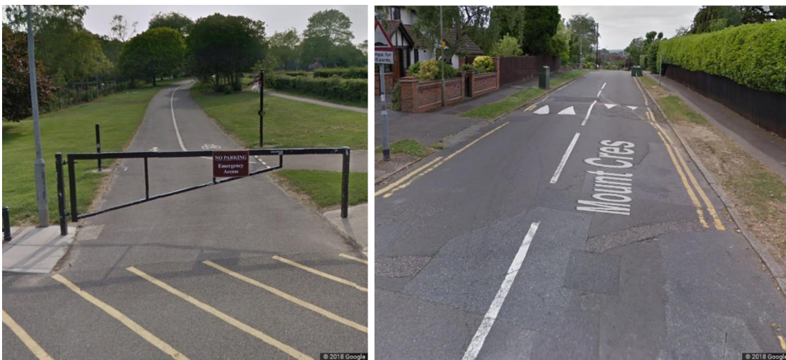
Figure 4.4: King George's Playing Field cycling route (left: segregated footpath/cycling track through King George's Playing Fields, right: on-road cycle lane on Mount Crescent)
