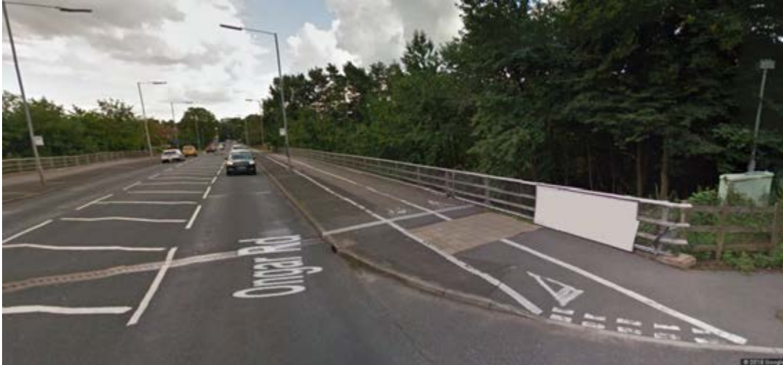
Figure 4.3: Ongar Road cycling infrastructure over A12 facing south
