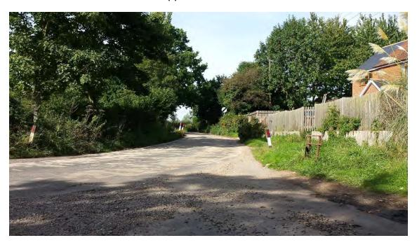
This surfacing has been installed to provide an increased skid resistance on the bends and as there are not any personal injury collisions recorded at either bend it appears to be working.
