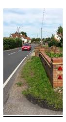
This is wall is set back 1.3m from the carriageway and although this does provide a small refuge area for pedestrians this is below the recommended minimum width of 1.5m
