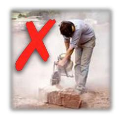
Dust is generated from these materials during many common construction tasks. These include cutting, drilling, grinding and polishing. Some of this dust is fine enough to get deep into lungs. The fine dust is known as respirable crystalline silica (RCS) and is too fine to see with normal lighting. It is commonly called silica or silica dust.
