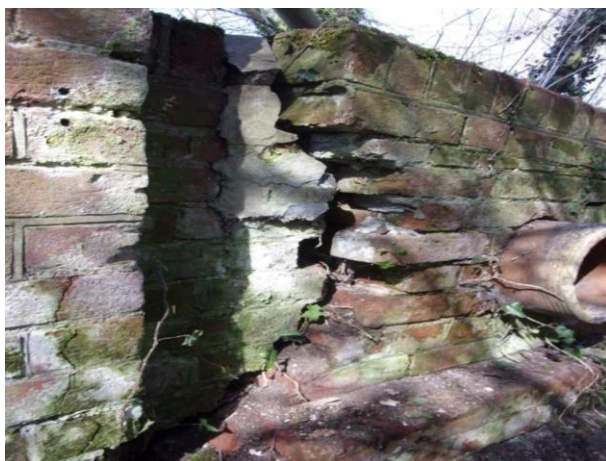
Above - Image 5: North-east wingwall
