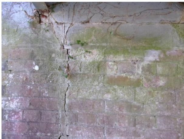
Above - Image 4: South Abutment
