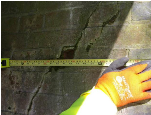
Above - Image 3: North Abutment
