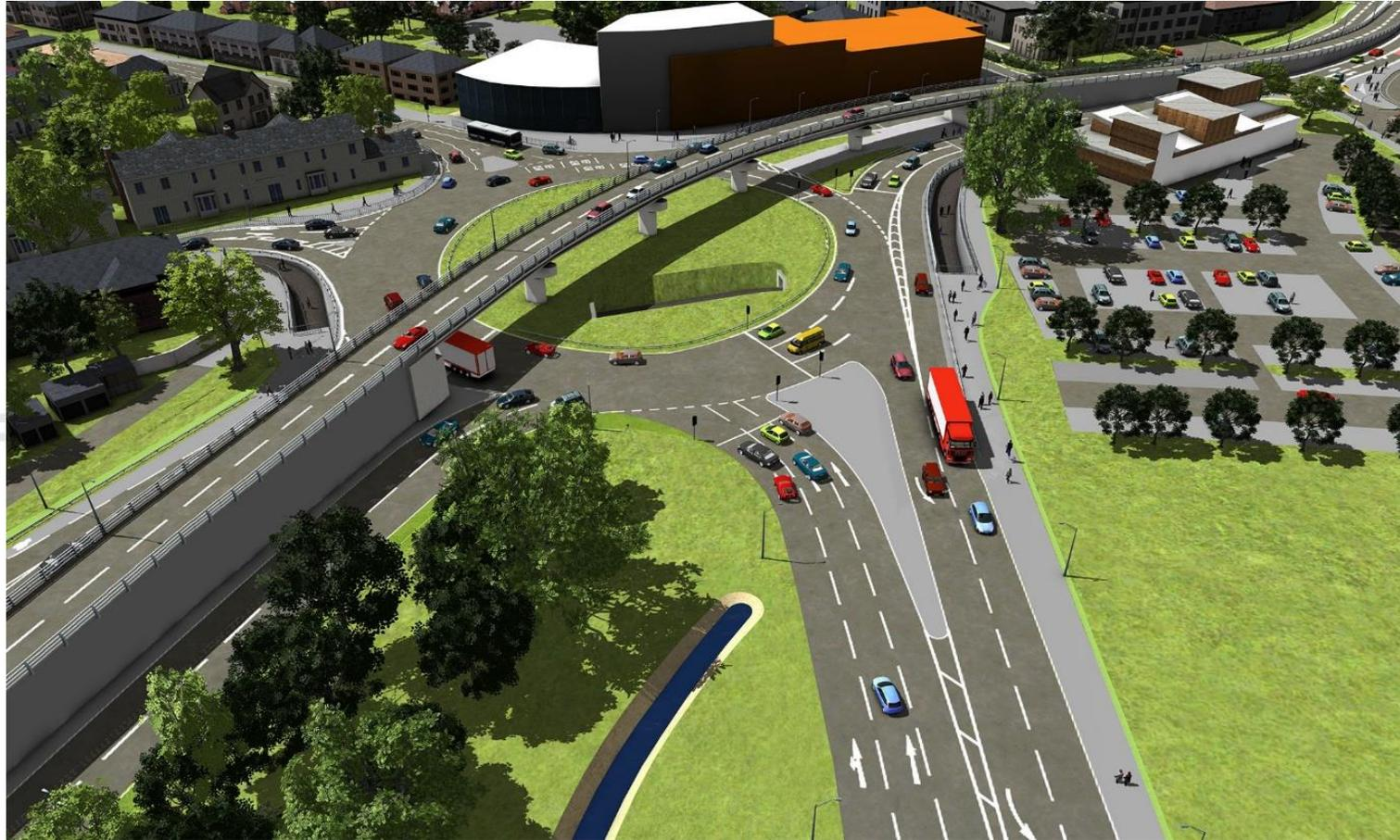
A new two-way flyover allowing a significant amount of traffic to travel to and from Parkway and Essex Yeomanry Way in both directions.
