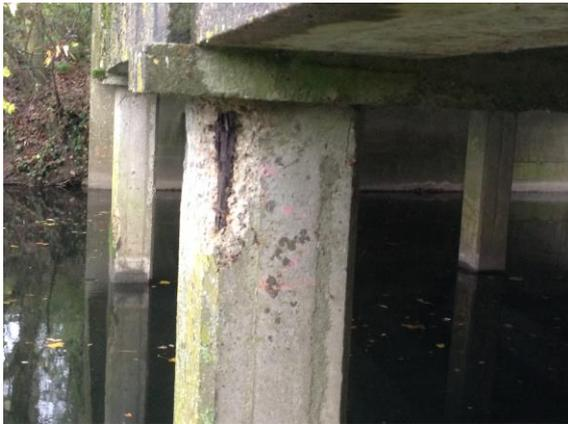
Photo 4. Localised spalled concrete
