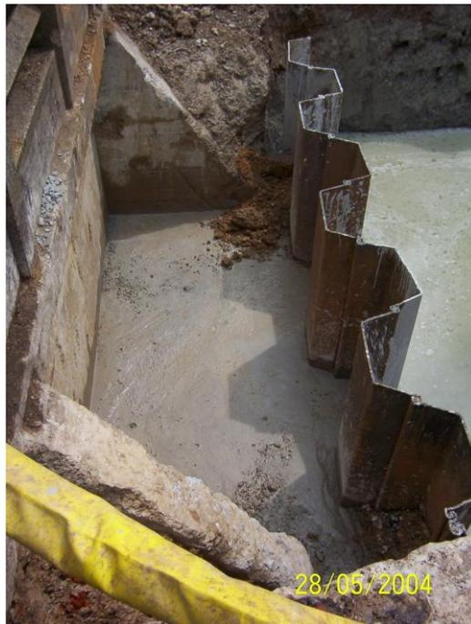
Photo 3. View of southern abutment sheet piling construction details (2004)
