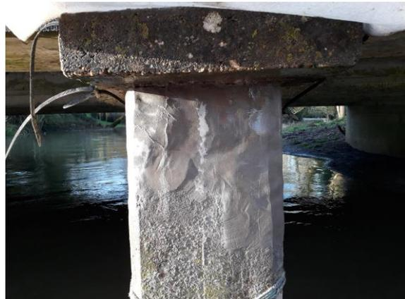
Photo 5. Completed concrete repair
