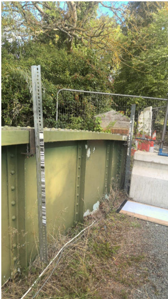
Figure 6 Typical 500mm barcode staffs clamped to the top flange, set vertically
