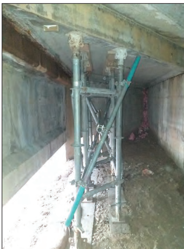
Figure 2: Interim Propping System (North-East Footway Slab)
