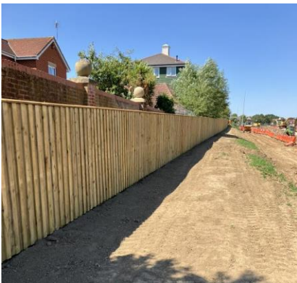
Section of acoustic fencing installed along the site boundary on Northern approach Road
