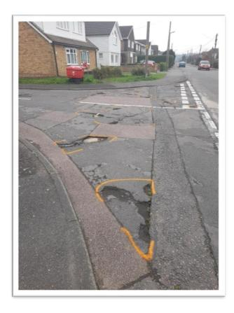
**Example 4** - Carriageway patching: various patches at different locations. Estimated completion is 1 to 2 hours per patch. One pothole/patch under give and take traffic management on a local road is estimated to take up to 1 hour per patch.
