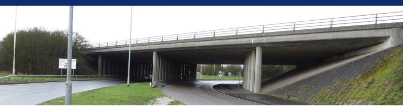
Arrangements have been made to refurbish this four span bridge and install new vehicle safety barriers known as a vehicle restraint system (VRS) as well as inspection platforms to support future surveys.
