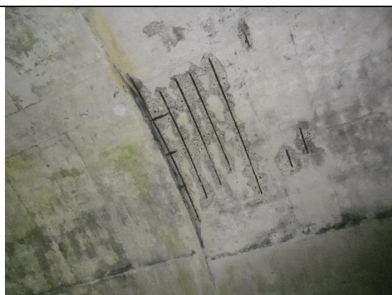
Spalling Concrete
