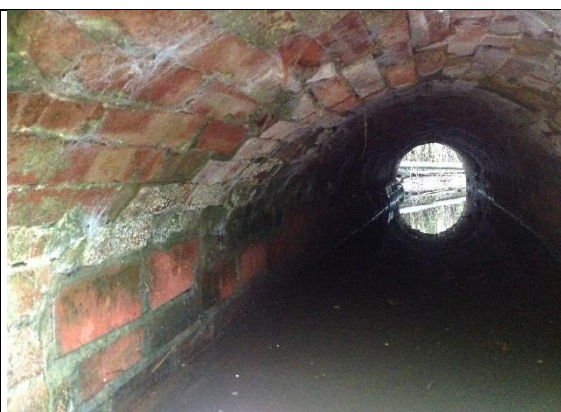
Bulging at crown of arch
