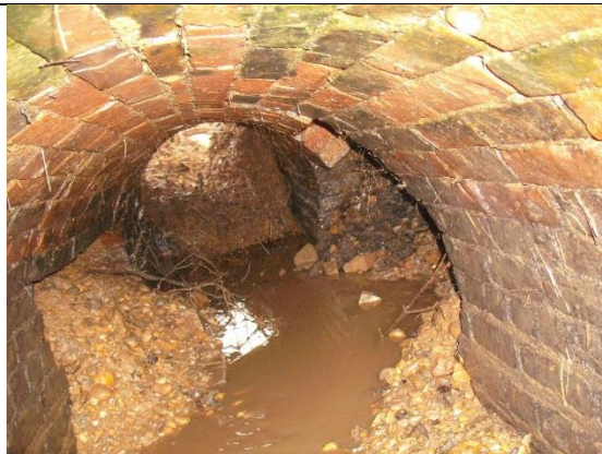
Backfill washed away
