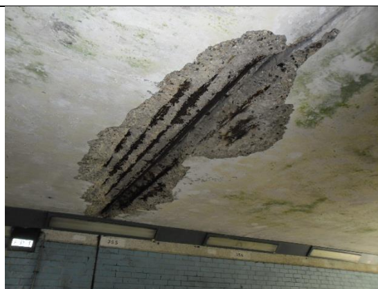
Spalled Concrete
