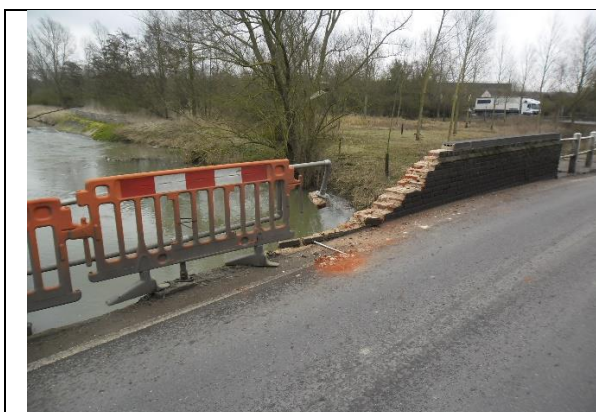
Parapet damage due to RTA
