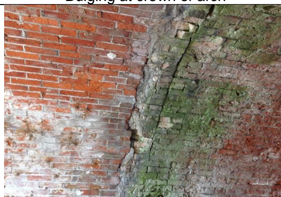
Cracked and spalling brickwork
