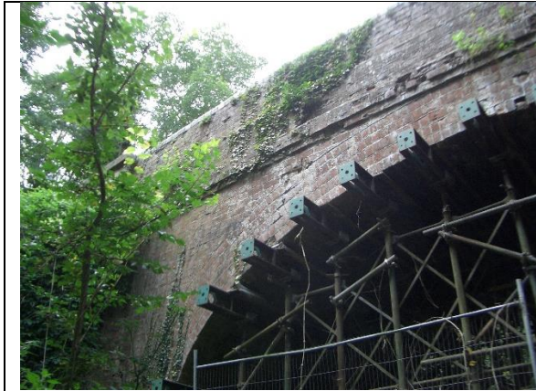
Setting up the propping system under arch
