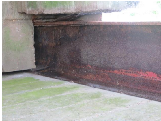
Delamination of beam
