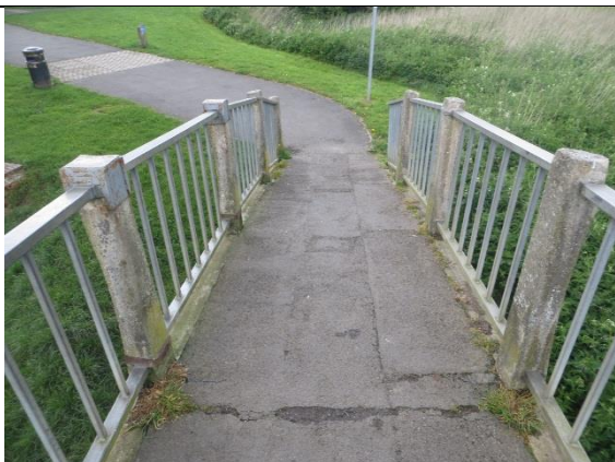
Footway surfacing and joint issues
