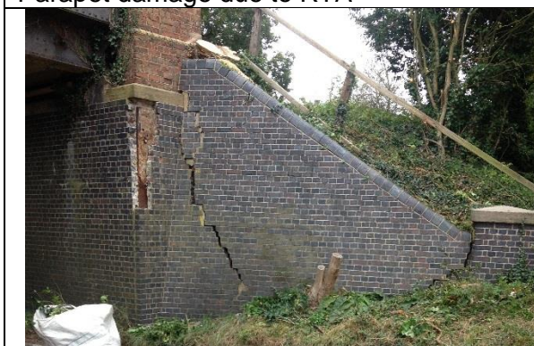
Badly cracked wingwall
