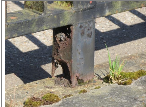
Rusting at base of parapet post
