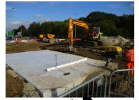
the roundabout have been removed and traffic island areas have been replaced with full road construction. This will allow more room for traffic management. The attenuation tank system has been fully installed together with much of the associated deep drainage.
