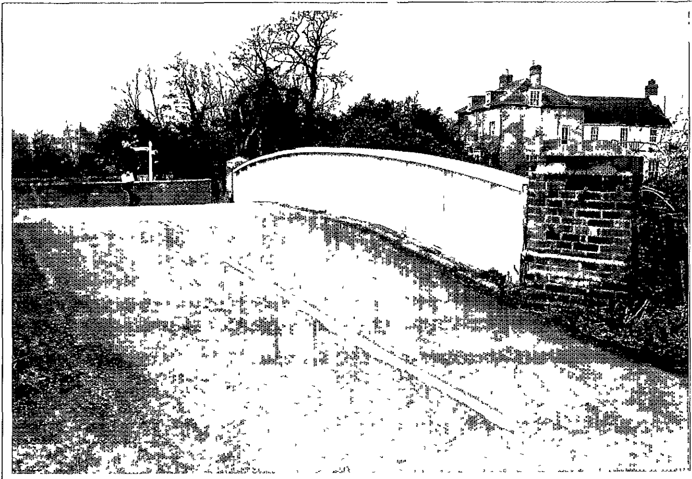
PLATE 3 VIEW FROM NORTH
