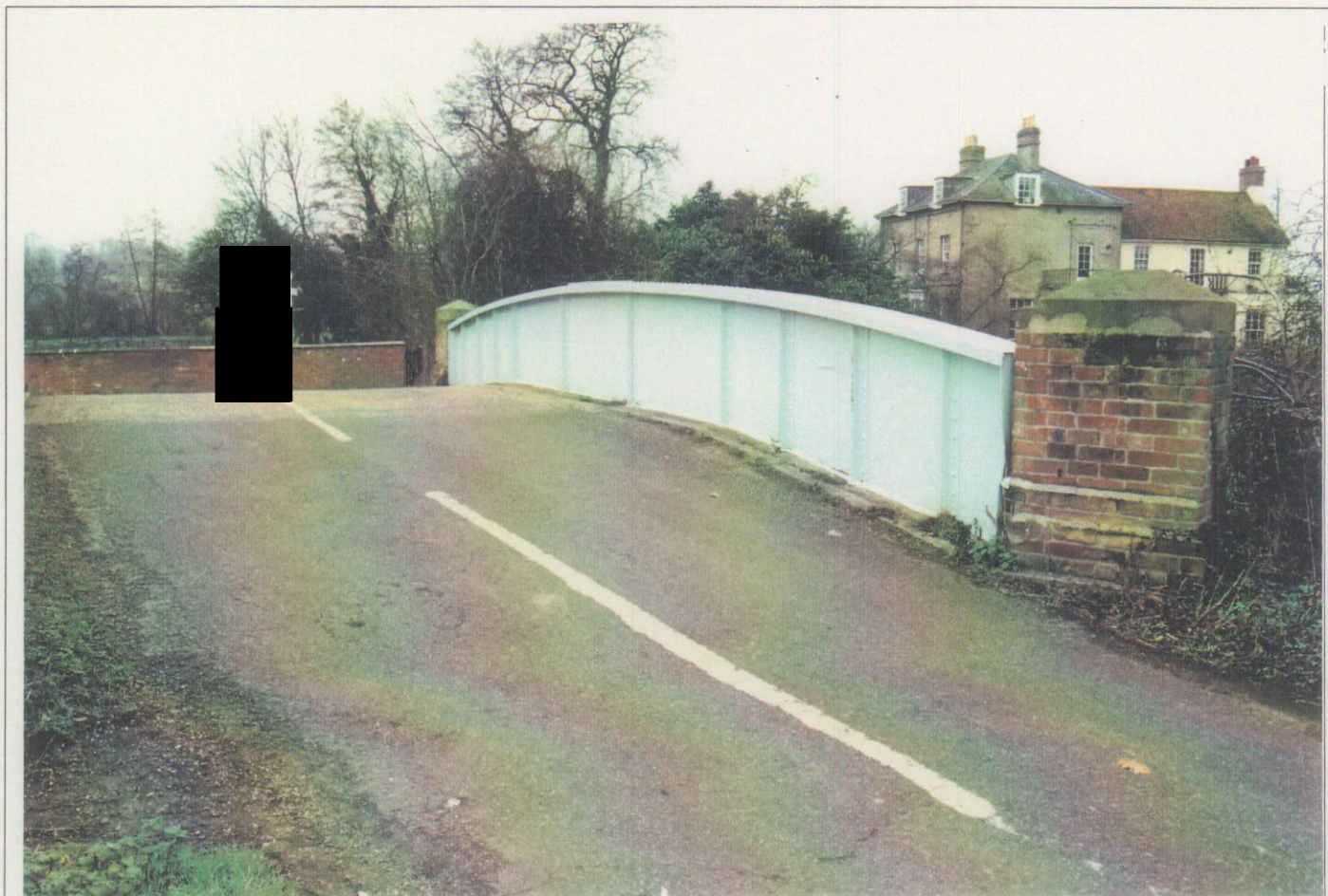
PLATE 3 VIEW FROM NORTH
