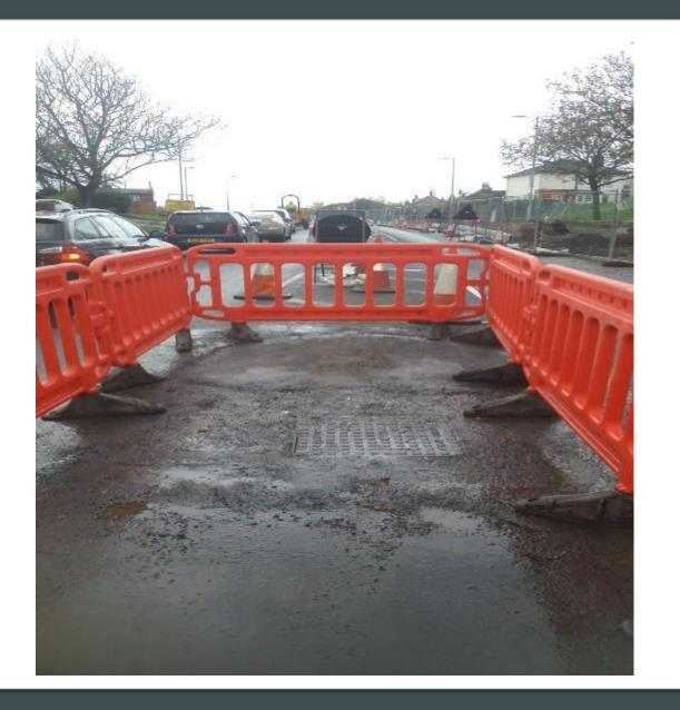
Traffic Island having Tarmac laid on St Andrews Avenue East of Harwich road roundabout. This is to enable traffic to run in the centre lane Heading Eastbound whilst works in Construction zone 1A continue.
