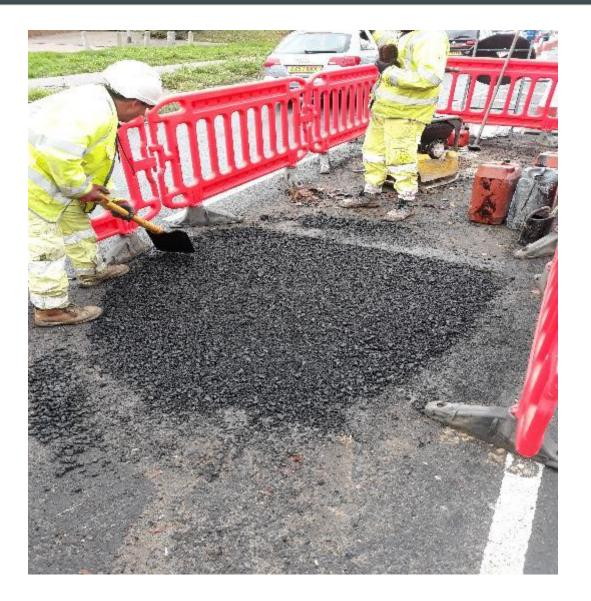
Traffic Island having Tarmac laid on St Andrews Avenue East of Harwich road roundabout. This is to enable traffic to run in the centre lane Heading Eastbound whilst works in Construction zone 1A continue.
