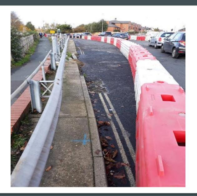
Traffic management in place on Ipswich road roundabout to facilitate the Hoarding works and trenching to be undertaken in this area.
