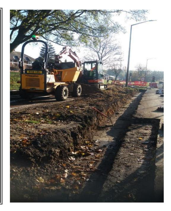
Construction zone 1A. Backfilling of sub layers for new kerb line to be laid.
