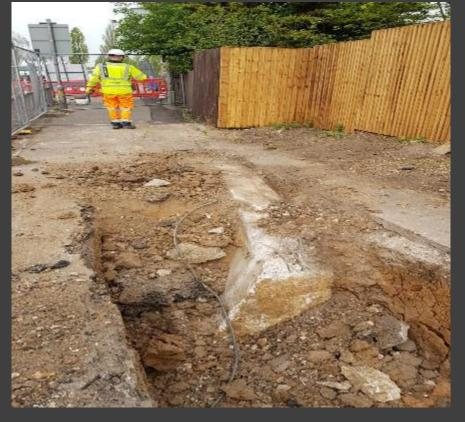
UKPN/BT being trenched and ducting laid around the footpath from Ipswich Road North to Cowdray Avenue
