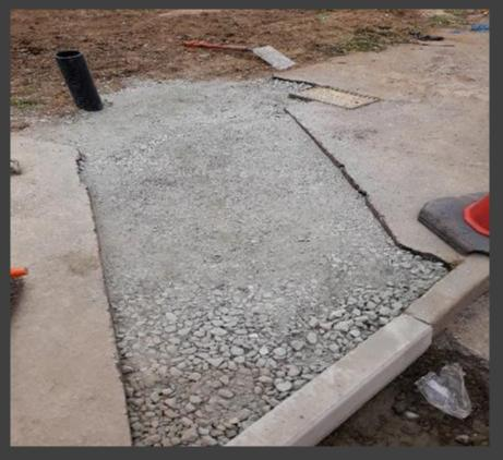
UKPN being trenched and prepped for ducting to be laid across Harwich Road South & into the Compound
