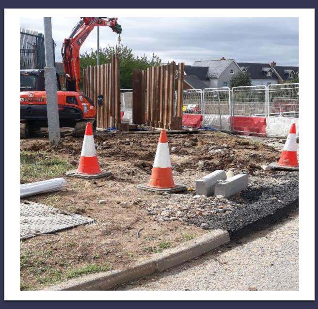
Sheet piles being installed for Manhole 7 at the corner of Homebase.
