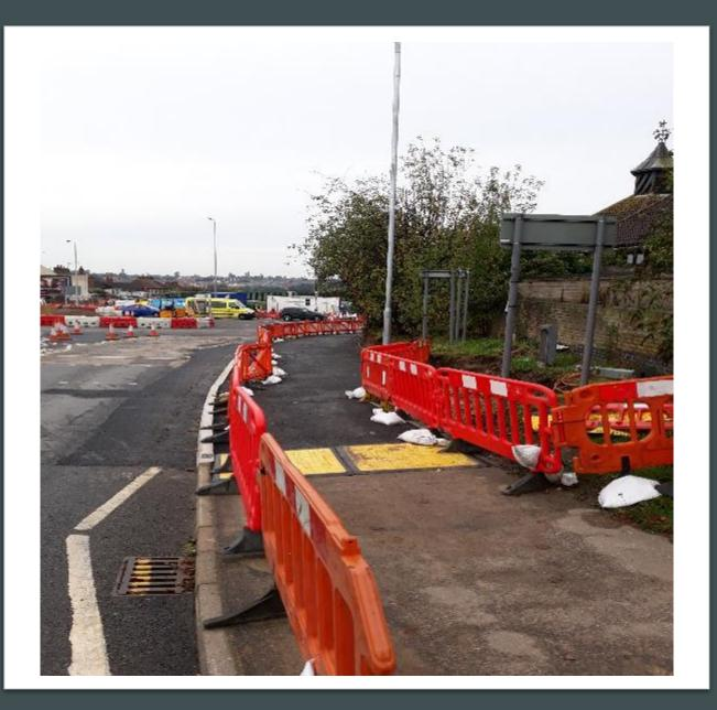
Construction zone 1B. Footpath resurfaced to base level and reopened.
