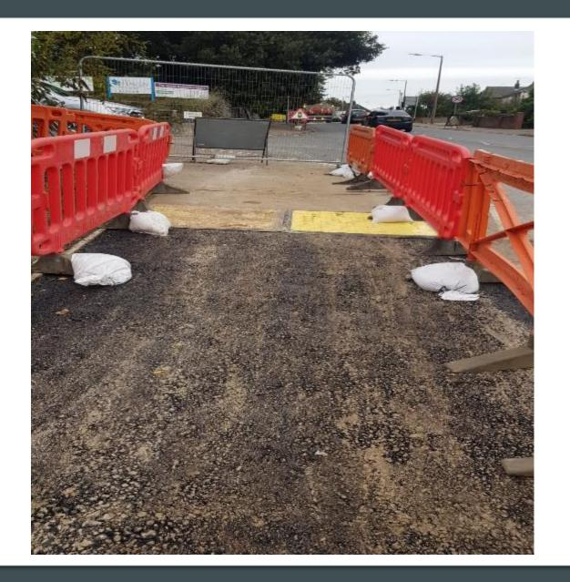
Construction zone 1B. Footpath resurfaced to base level ready to be reopened.
