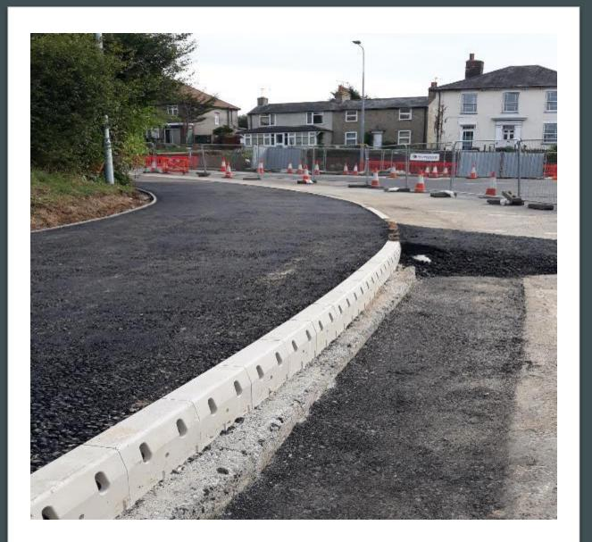
Construction zone 1B. Footpath Resurfacing works to get this section of footpath reopened. Construction zone 1B – St Andrew's Avenue. Footpath Resurfacing works.
