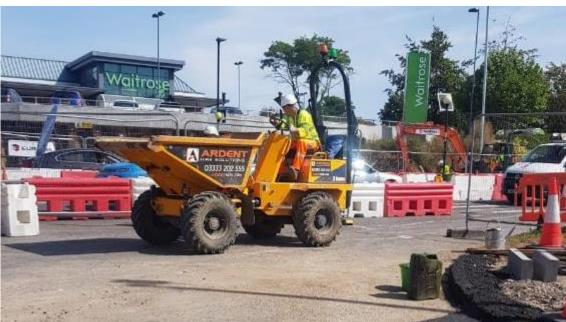
Ipswich Road South- Backfilling and reinstating excavations for Anglian Water Diversions.
