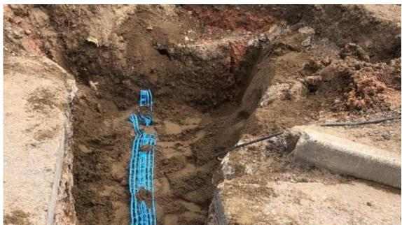
Ipswich Road South-Backfilling and reinstating excavations for Anglian Water Connections/Diversions.
