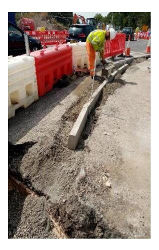
Marking out and trenching across St Andrews Avenue for ducting to be installed ready for the new pedestrian controlled signal crossing.
