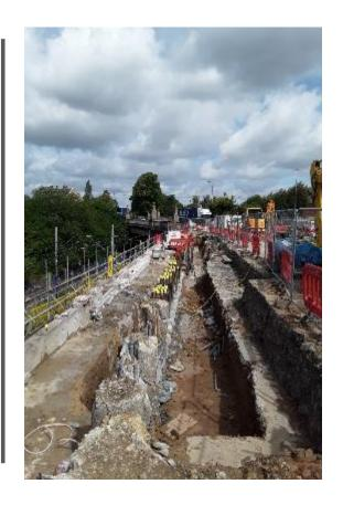
Retaining wall dig, exposure of the piles and removal of the retaining wall in construction zone 2D.
