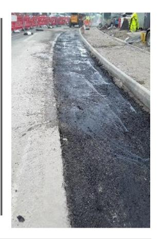
Kerb/edging completion and asphalting of footpath and carriageway in construction zone 2B.
