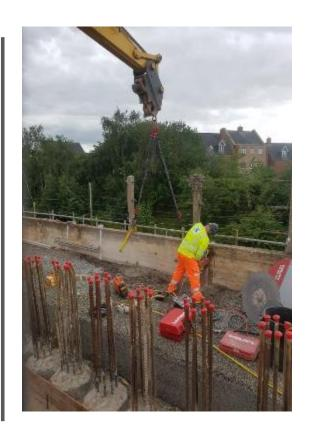
Retaining wall dig, exposure of the piles and removal of the retaining wall in construction zone 2D.
