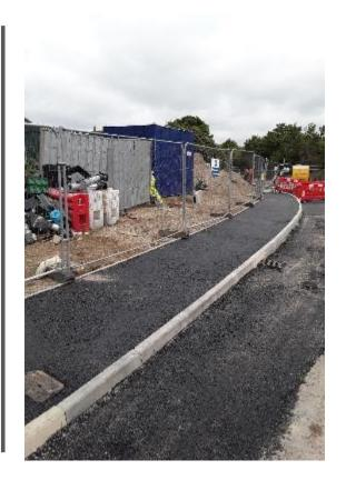
Kerb/edging completion and asphalting of footpath and carriageway in construction zone 2B.
