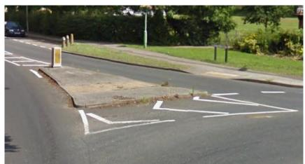
Image 8: Example of flared road marking at roundabout, reducing roundbaout circulatory.
