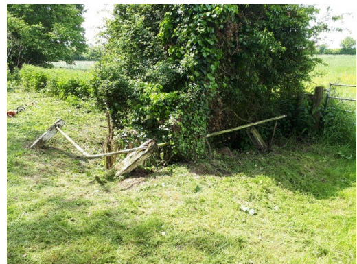
Hempstead railings- before
