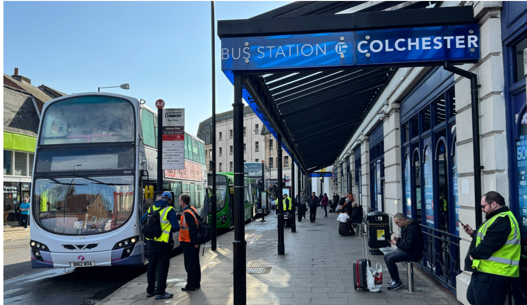
Existing Colchester Bus station at Osborne Street
