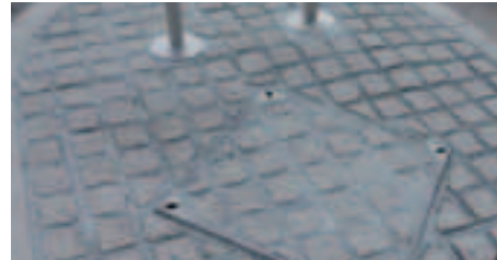
Cover should have been aligned with paving pattern or maybe a round cover used
