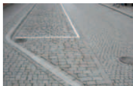
Example of poor use of white lines imposed on a parking space already defined by using different block sizes
