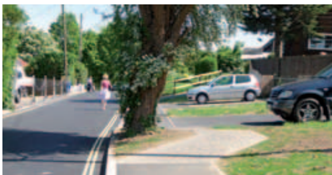
Permeable paving as used here on a new footway around an existing tree in Maldon.
