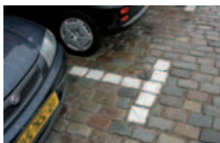
Example of a designed approach to line marking related to the surface material used
