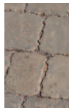
Permeable paving as used here on a new footway around an existing tree in Maldon.
