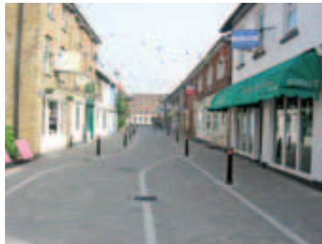
Shared surface in Brentwood using tumbled blocks with the carriageway marked by a different colour banding
