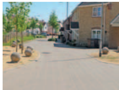
Shared surface at Beaulieu Park, Chelmsford using block paving and granite kerbs
