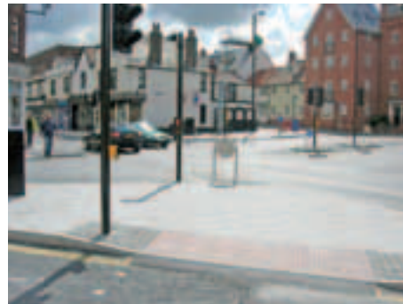
Brentwood High Street using reconstituted granite paving
