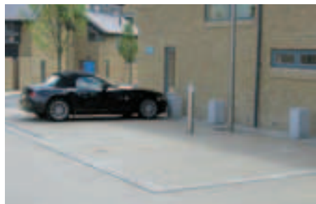
Above: Parking spaces defined in bound gravel by the use of granite setts. Harlow, Essex
