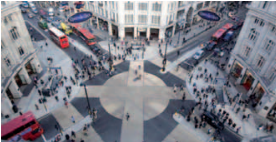
Example of a recent innovative remodelling of a main junction at Oxford Circus, involving guard rail removal and free flow pedestrian movements
