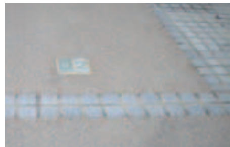
Above: Parking spaces defined in bound gravel by the use of granite setts. Harlow, Essex
